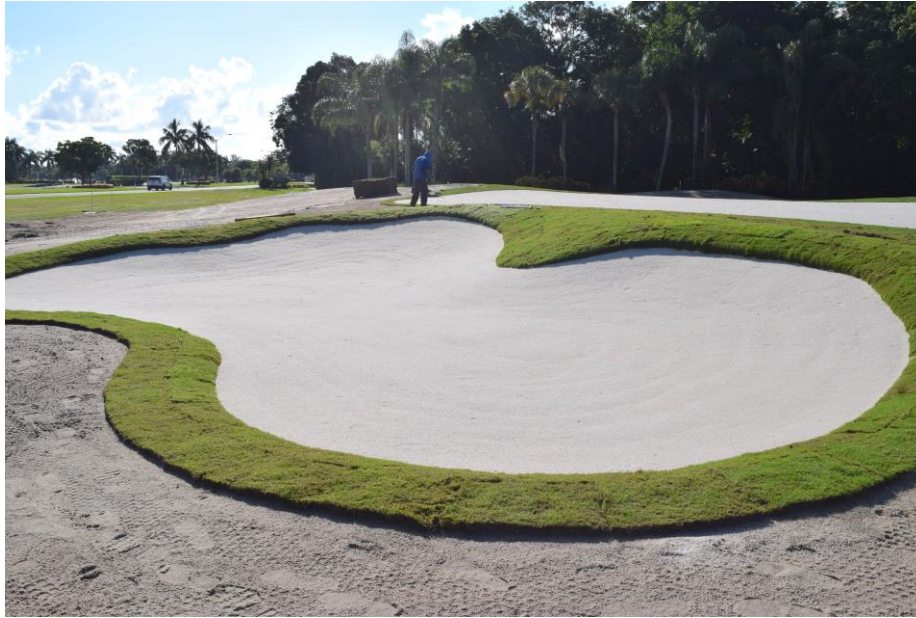
South Course bunker renovation in progress (photo by Jan Bel Jan, ASGCA)
